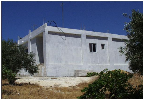
Nidal Abu Sitta's house threatened with demolition.
